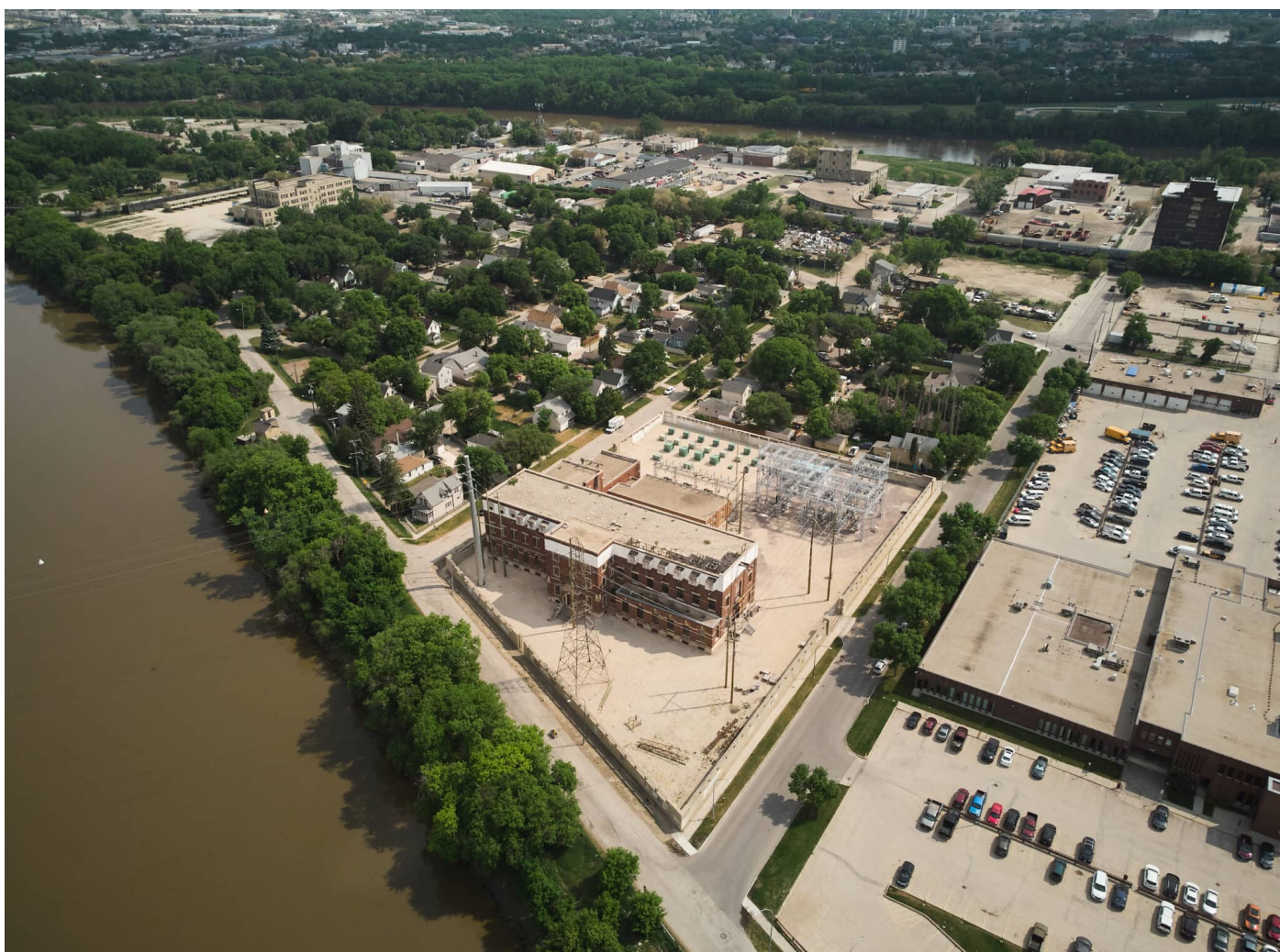
Two historic energy buildings — the vacant Rover Avenue electric terminal (left) and a former coal gasification plant now owned by Manitoba Hydro — sit right against the Red River. A benzene plume has been slowly flowing from this block into the river sediment. Photo: David Lipnowski / Winnipeg Free Press
