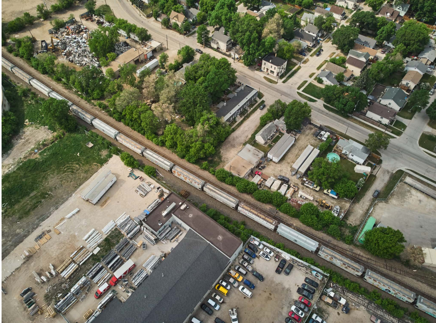
Heavy manufacturing, active rail lines, vacant lots, social housing and some of Winnipeg's oldest homes are crowded into just 1.8 square kilometres in the Point Douglas neighbourhood. Photo: David Lipnowski / Winnipeg Free Press
